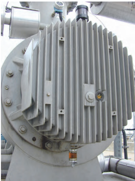
BOS Drain Bottle/BS&W Bowl on Centrifugal Pump running on Royal Purple Synthetic Oil
